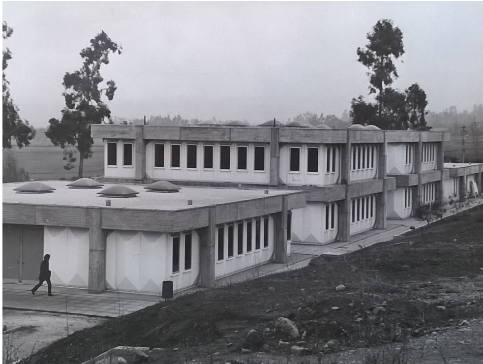
Figure 4. Modular coordination between structure and elements of enclosure in Normal School of La Reina (1969), Santiago of Chile. Fuente: PUC Archive.
