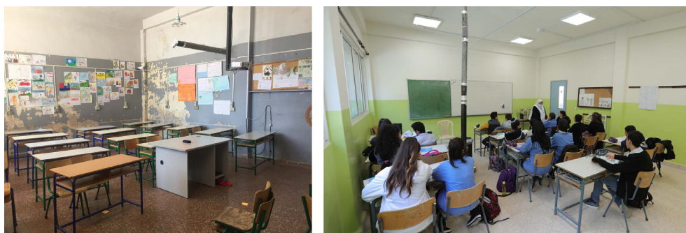
Figure 1. The status of the indoor spaces in Amatour public school before and after the renovation. GIZ Lebanon, education program, 2018.
