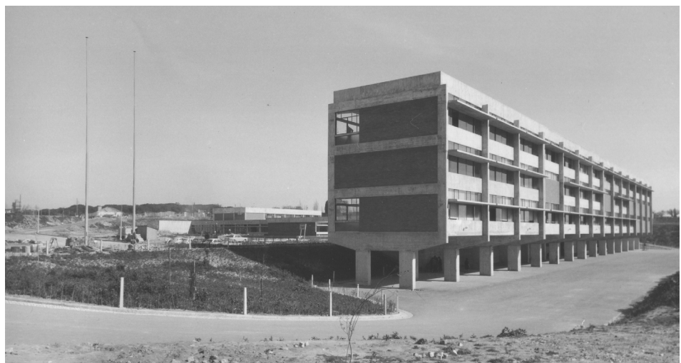
Figure 6: View of the south façade, with the shades above the classroom windows.
