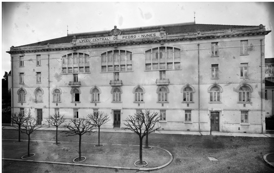
Figure 1: Liceu de Pedro Nunes (1908-1911), Lisbon. Main façade.
