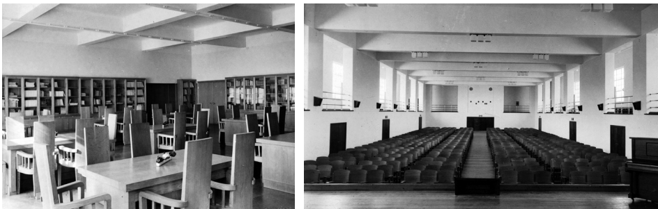
Figure 7: Liceu de D. Filipa de Lencastre (1932-1940), Lisbon. Horizontal structural elements (beams and floors) in reinforced concrete.
