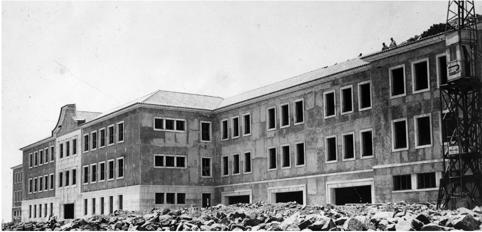
Figure 3: Liceu de D. João de Castro (1944-1949), Lisbon. Main building under construction.
