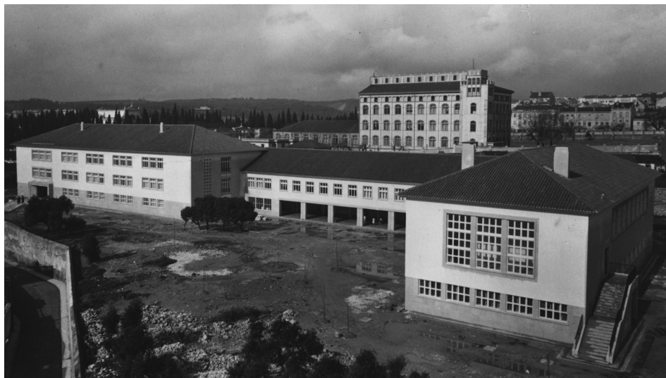
Figure 3: Escola Industrial Feminina Josefa de Óbidos after its construction: there is a visible contrast between the predominantly horizontal large glazed openings and the tiled roof with eaves, highlighting the compromise between the construction based on the use of traditional methods and the features suggesting a more modern image, as established in the Standardised Preliminary Design.
