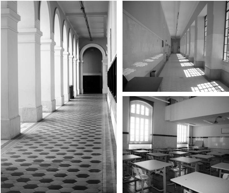
Figure 2: . Gallery leading to the courtyards; Corridor providing access to the classrooms on the first floor; interior of a classroom.
