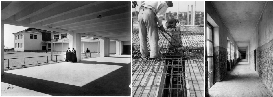
Figure 4, Figure 5 e Figure 6: Liceu de Sá da Bandeira (1939-1943), Santarém. Horizontal structural elements (beams and floors) in reinforced concrete and vertical structural elements made of masonry.
